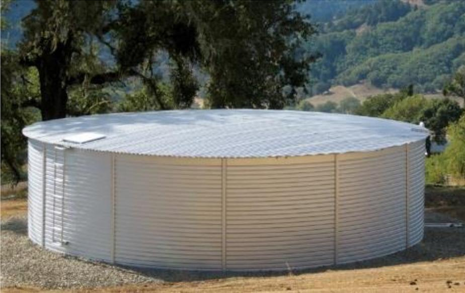
The metal dome roof offers strength and flexibility for new and existing tanks
