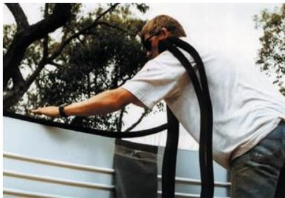
*Gluing Presstite to top rim of tank*
