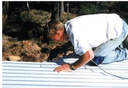
*Trimming roof sheets to tank diameter*
