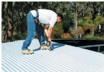
*Laying and fitting steel roof sheets*
