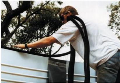
*Gluing Presstite to top rim of tank*
