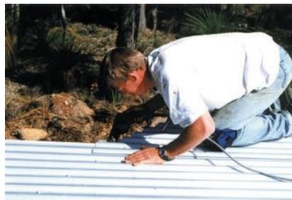
*Trimming roof sheets to tank diameter*
